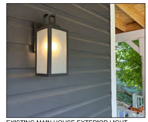
EXISTING MAIN HOUSE EXTERIOR LIGHT
